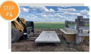
**INSTALL:** Set into place (utilizing the built-in chain system) with a loader and chains, pallet forks, the bale bed on your pickup, or a crane. We recommend filling in any large gaps between the pad and your waterer.
