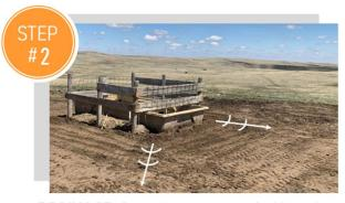
**DRAINAGE:** Create drainage spot, preferably on the low side of tank. We use a skid steer to dig a shallow ditch. This is to allow the majority of rain water or, if the float breaks, overflowing water to drain away from the tank and Stock Step.
