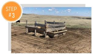
**PACK:** Pack dirt level with the bottom of the tank. Spread a layer of loose dirt or gravel on top of the packed dirt, approximately 2 inches is sufficient. Leave this dirt unpacked.
