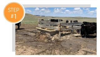
**PREP:** Clean out mudhole of mud, water, and slop. Scrape down berm and fill in mud hole, packing as you go. We use a skid steer to pack, driving back and forth with a scoop of dirt (for added weight), careful not to hit the tank.
